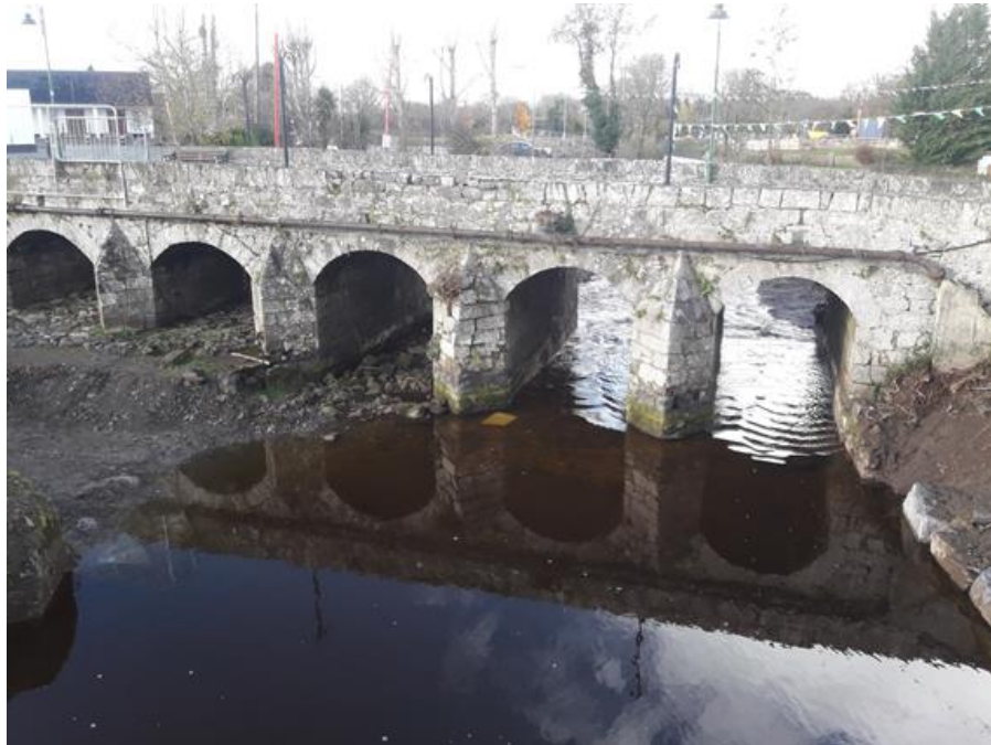
Figure 6; Regrading of Dunkellin complete
