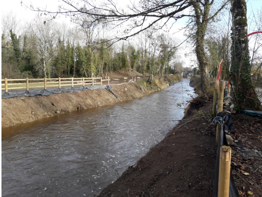
Figure 5; Regrading of Dunkellin complete
