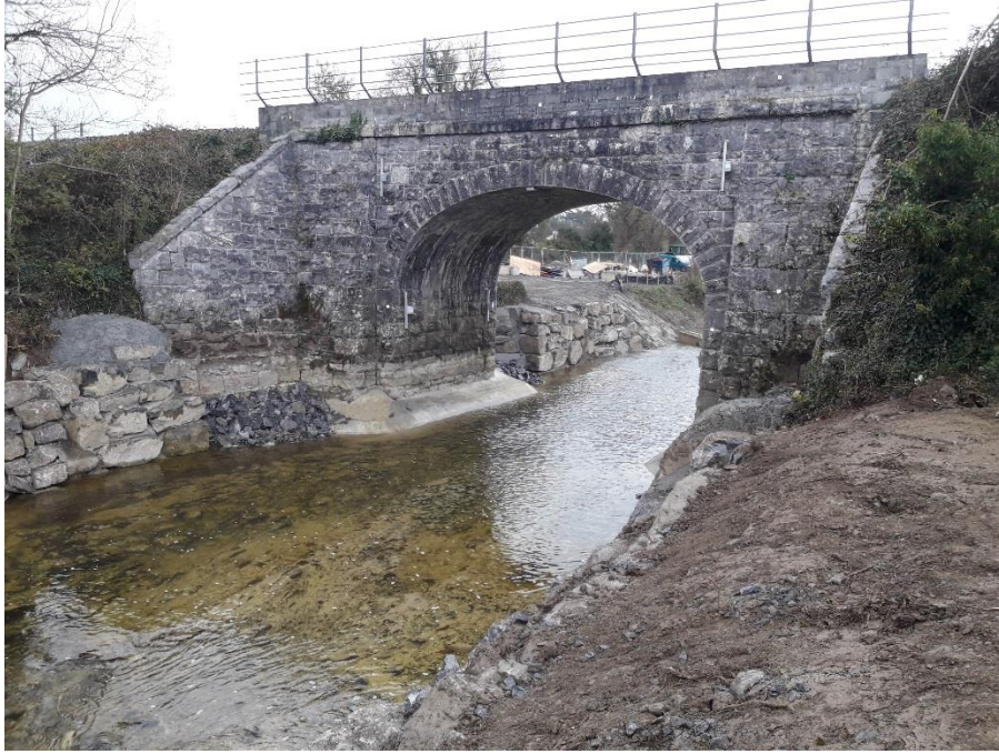
Figure 7; UB154 Railway Bridge
