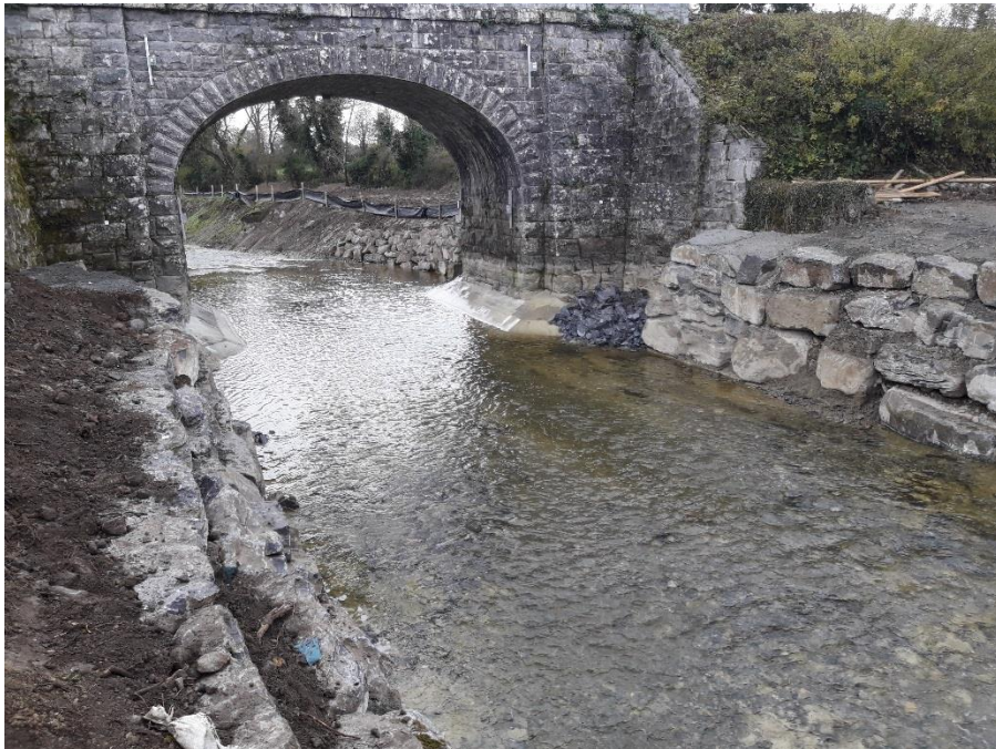
Figure 8; UB154 Railway Bridge
